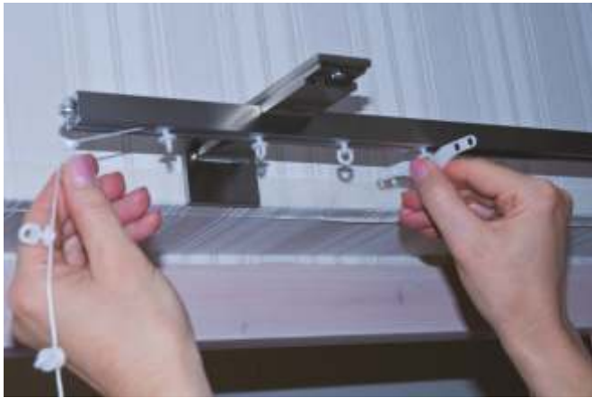
19 Insert the carrier cord in the curtain rail.
