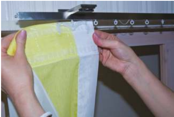
20 Insert the curtain into the carrier cord starting with the end-hook.
